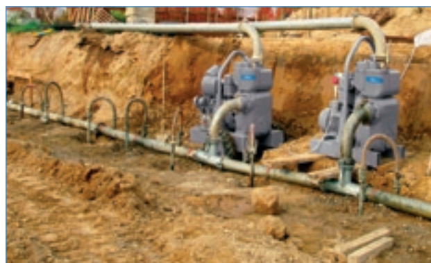
Wellpoint Vacuum dewatering
