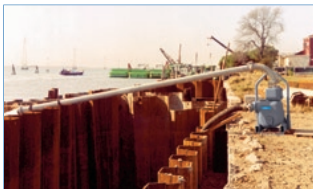
Construction site dewatering
