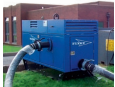
DWV Sewage by-pass pump
